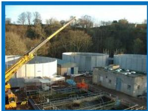
SBRs can be designed for continuous inflow or batch inflow. Both systems have their advantages and disadvantages but for a true batch system there is a requirement for a balancing tank in order to balance the flows out of the plant and prevent pulses of flow passing out of the works. The size of balancing tank required after the SBRs is dependant upon the instantaneous flow rate as indicated in the consent standard.
