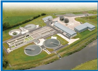
Lower ammonia levels require filters of greater than 1.8m depth and very often filters in series are provided to achieve the required loading rates. Either way trickling filters are susceptible to high peaks in ammonia passing through the system and causing high spikes in the effluent. They are however simple to operate and are highly dependable for carbonaceous removal and ammonia removal providing a reasonably smooth influent concentration is experienced.
