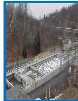
For sewage treatment, SBR size tends to be driven by hydraulics rather than biology on a sewage system particularly if the sewage is dilute. This means that it can be bigger than it needs to be for the biological load which obviously has a knock on cost implication and can mean that control of the biological system is difficult.
